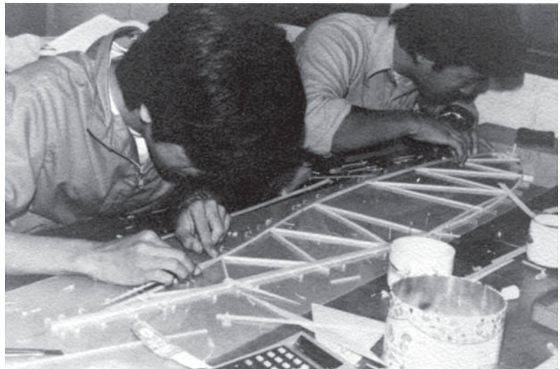
Assembly of a wing rib of the Stork
